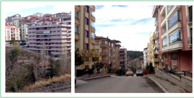
Figure 3. The regenerated built environment
