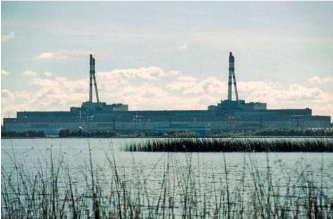
Fig. 14 The Ignalina nuclear power plant, the same reactor type as the one in Chernobyl. Source: Philipp Schmidt-Thomé 2003.
