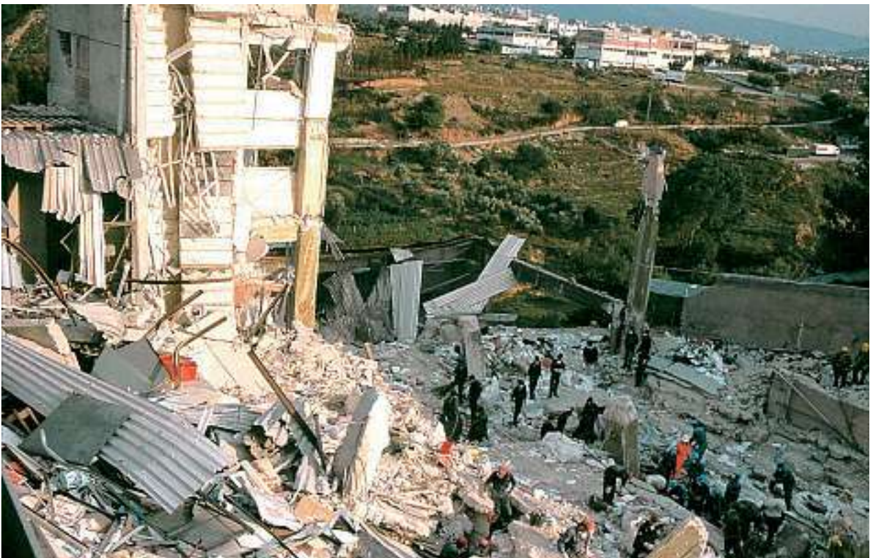
Fig. 3. Earthquake in Athens 1999. Source: Michael Fardis.
