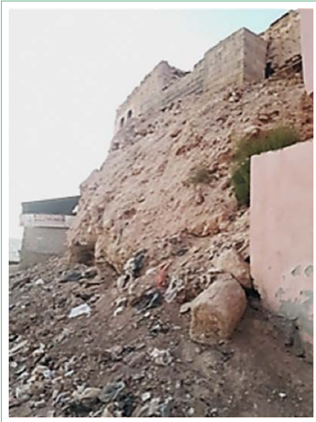
Figure 18. Landfill. The western side of the hill. Artificial elevation and the resulting subsidence (Photographed by the authors, 2018).
