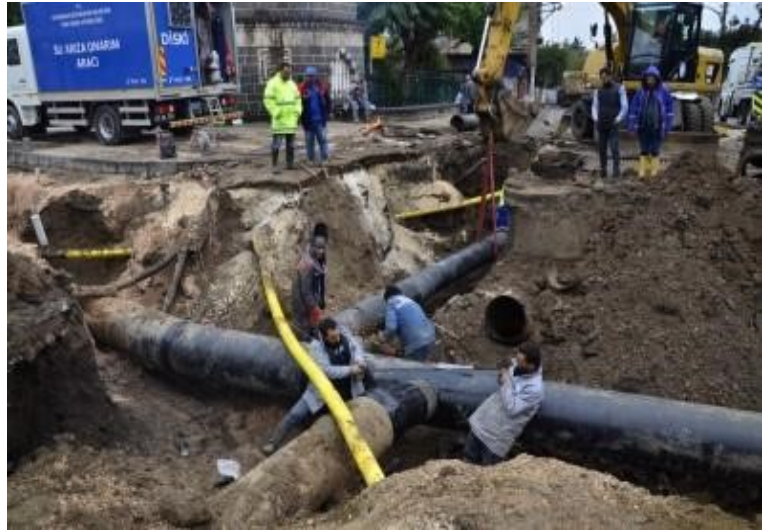
Deep and wide excavation area right in front of Urfa Gate
